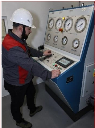
A pneumatic hydroelectric power station for hydraulic and pneumatic testing.
